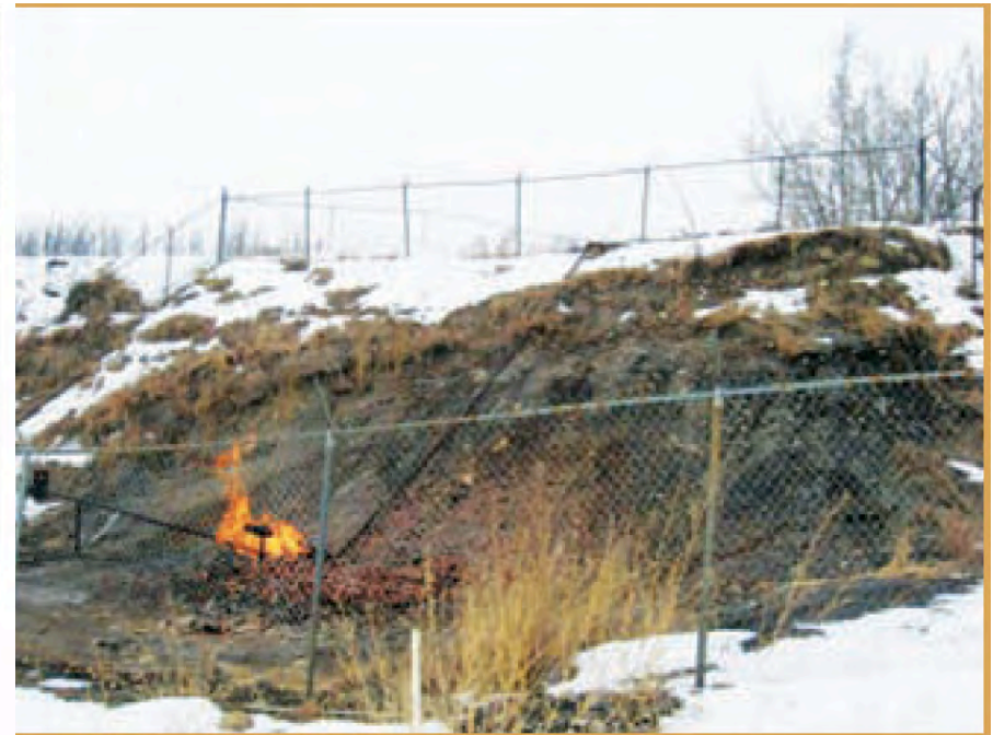
Gas well, leaking 1914-2010, Turner Valley, Alberta
